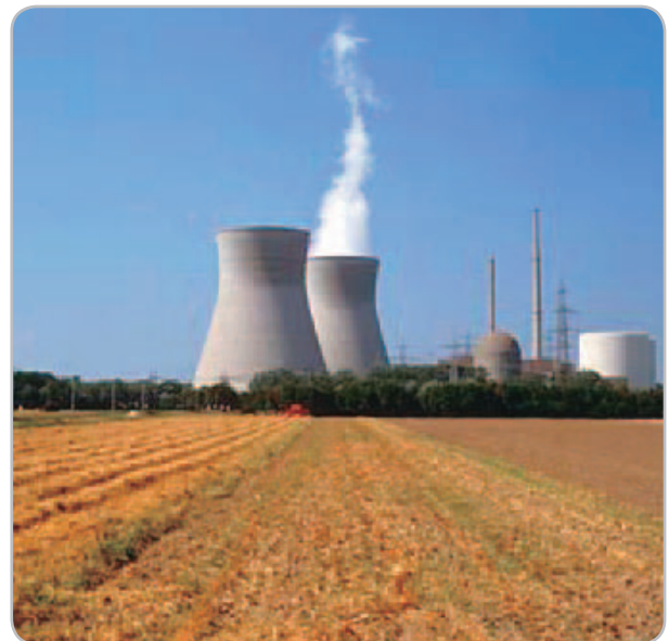
THE GUNDEMMINGEN NUCLEAR POWER PLANT IN GERMANY. SOURCE: ENCARTAMSN.COM
