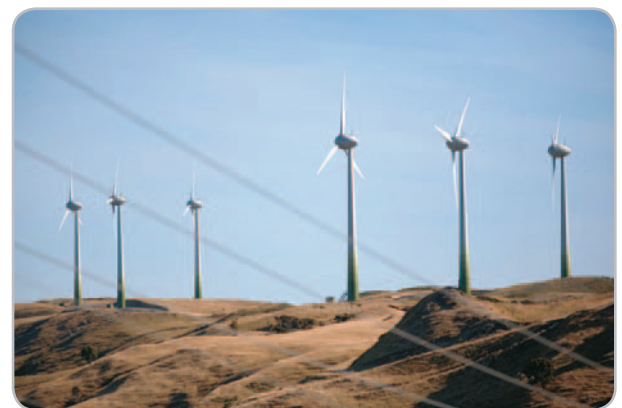
RENEWABLE ENERGY AT HAU NUI WIND FARM, WAIRARAPA SOURCE: GENESIS ENERGY
